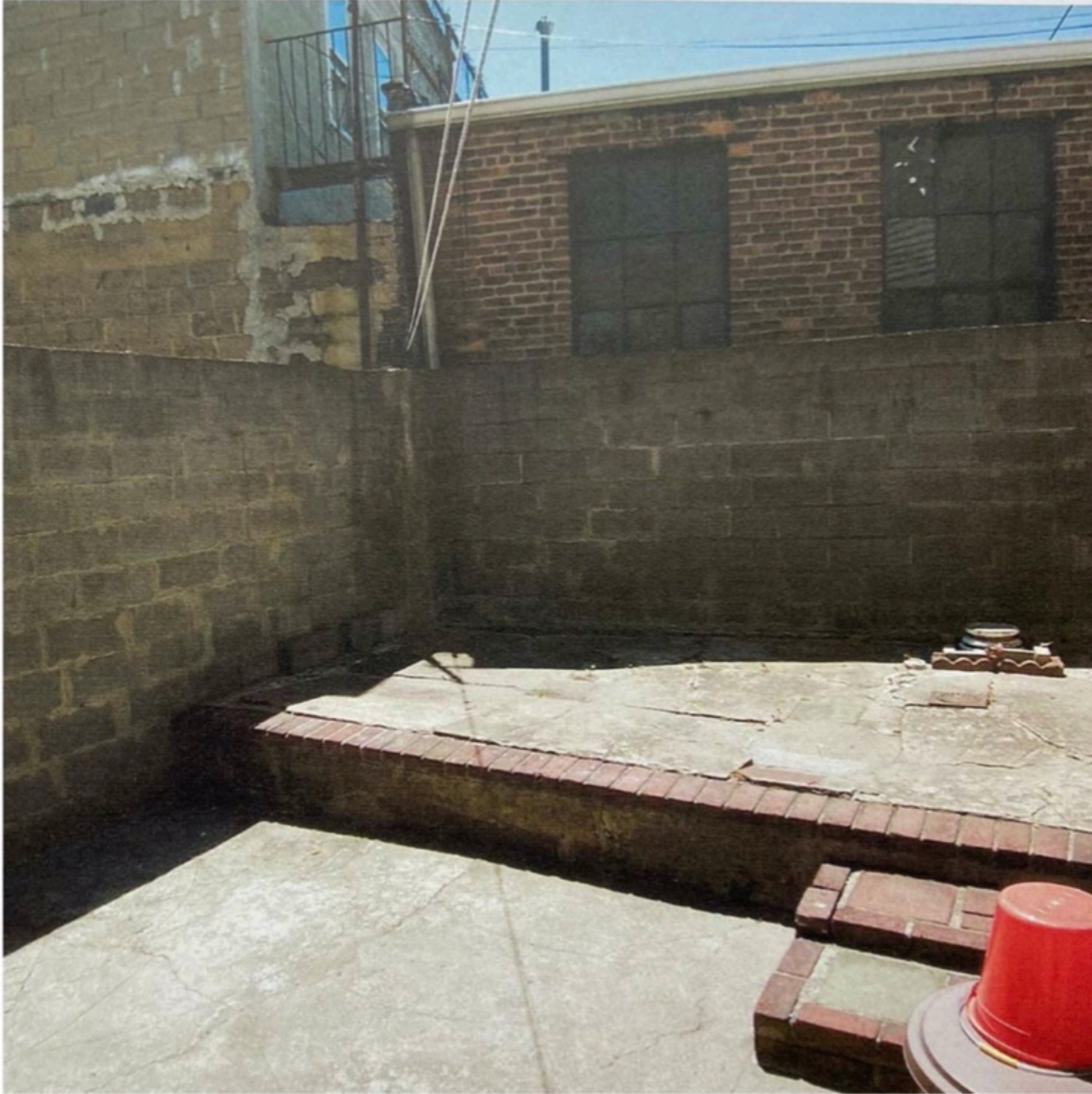
The outdoor lounge before the renovation. Photo: Greg Endries
